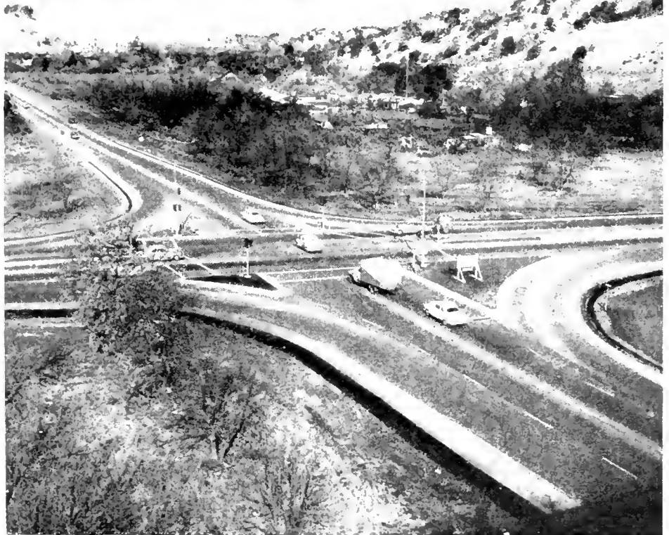
Two views of federal aid secondary county highway near Martinez. This section was constructed on a limited access freeway basis.
